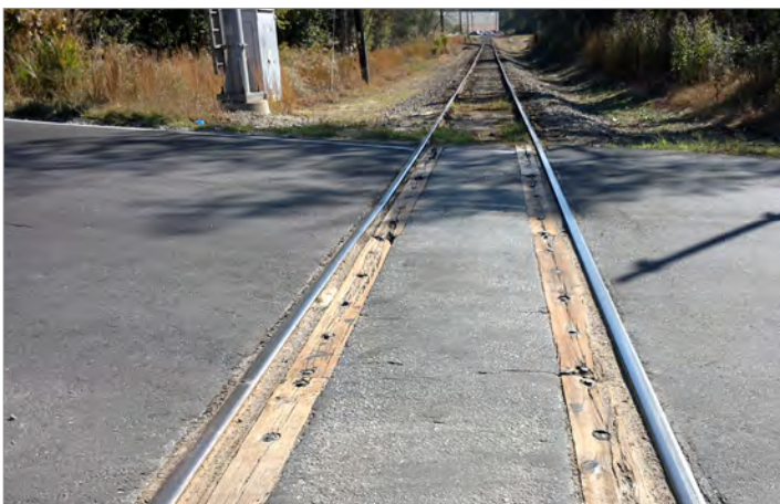
Cane Creek Road crossing before improvements
