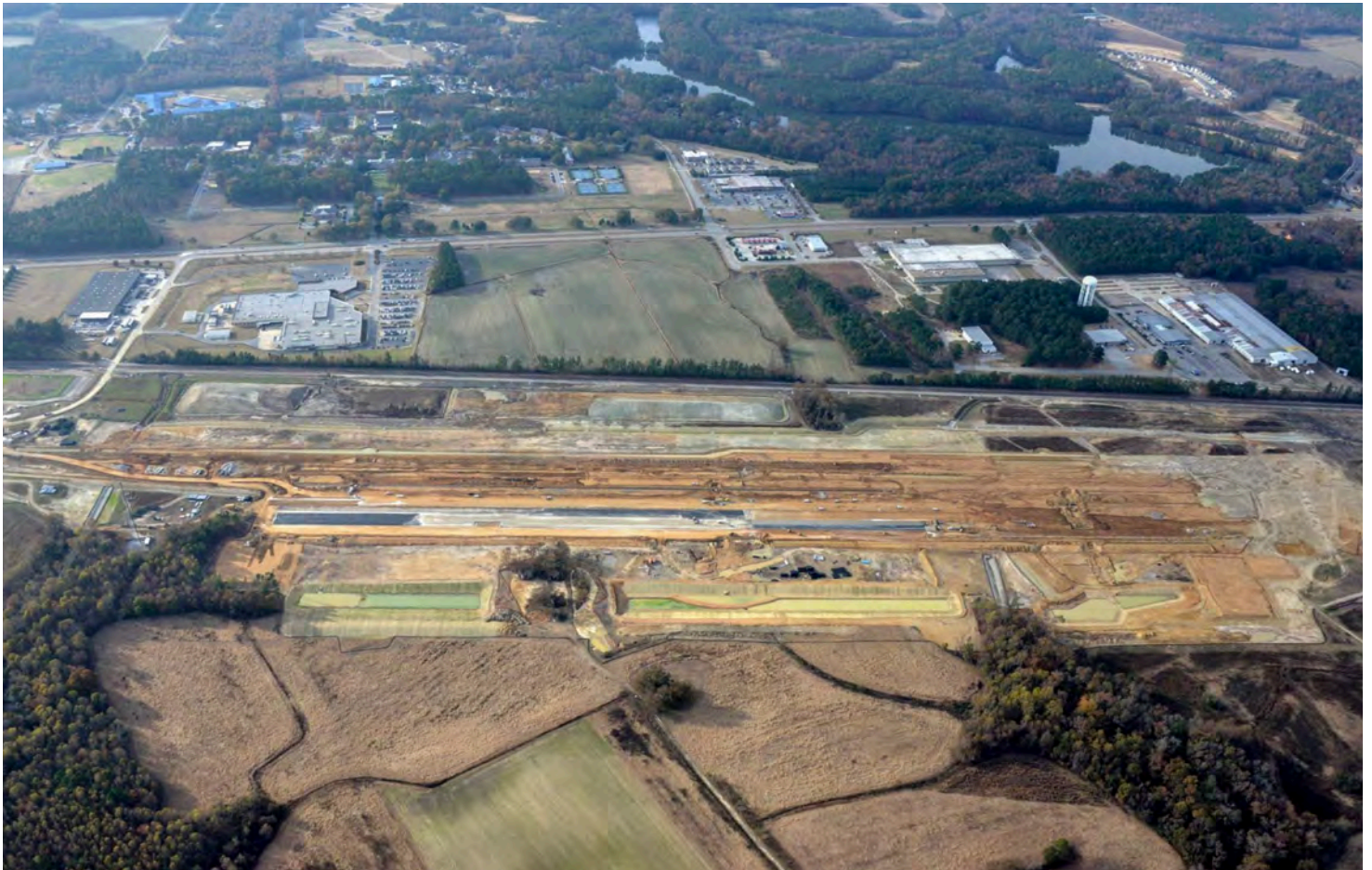
Aerial view of terminal site looking west
