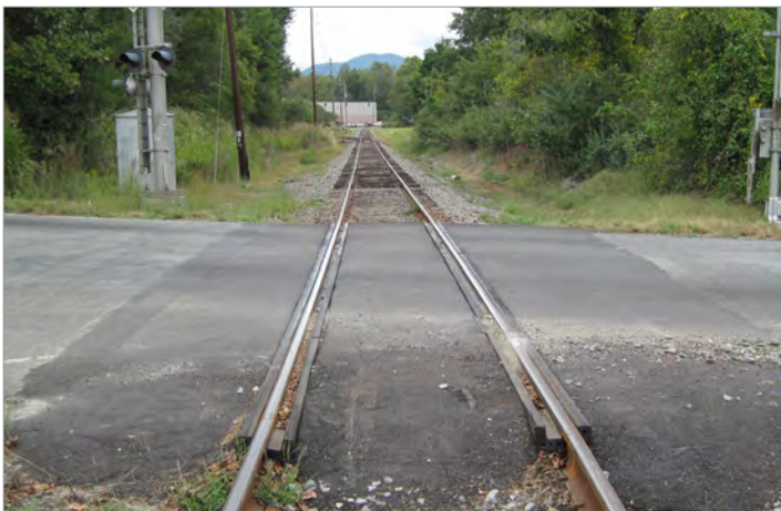
Cane Creek Road crossing after improvements
