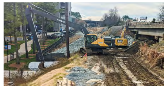
Retaining wall work by Bank of America Stadium
