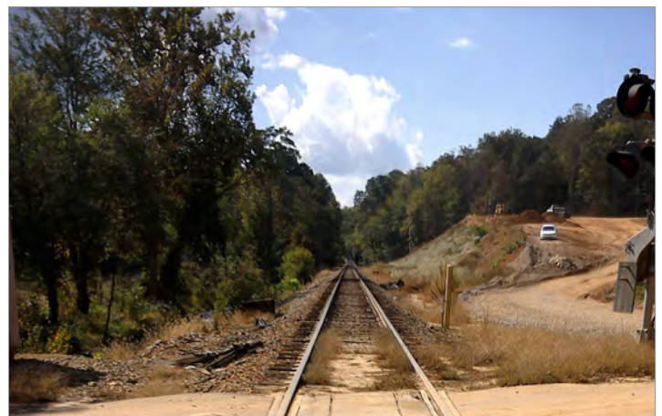
Hominy Baptist Church Road crossing before improvements
