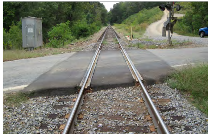
Hominy Baptist Church Road after improvements
