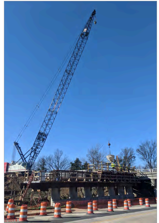
Pouring 4th Street bridge cap
